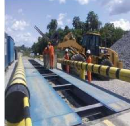
Weigh bridge foundation construction/installation@Gbaran ubie protection works LNG-SPDC
