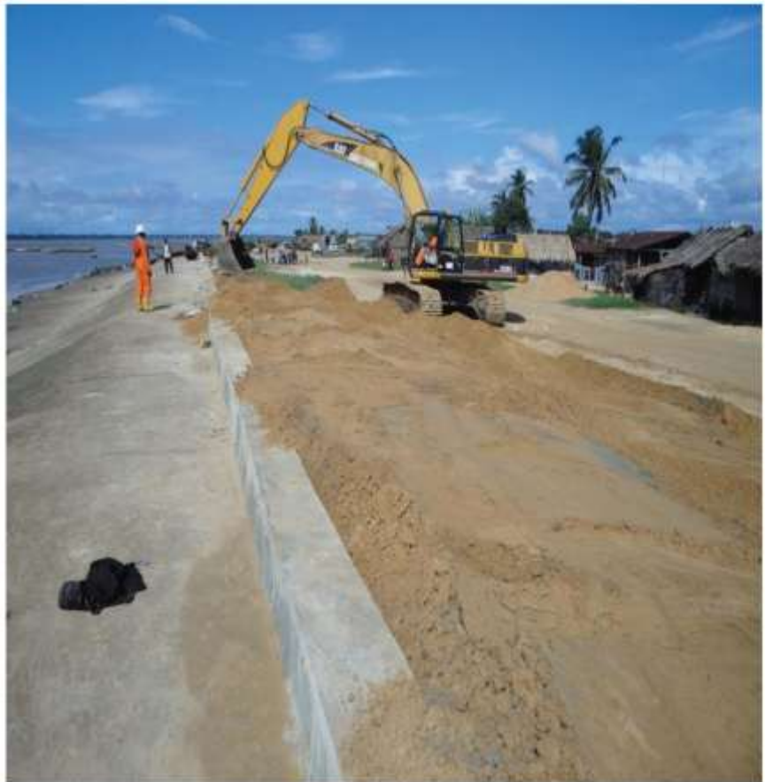
600m revetment construction (shore protection works) for SPDC at Ogu/agma, Forcados, Oe/ta Sate
