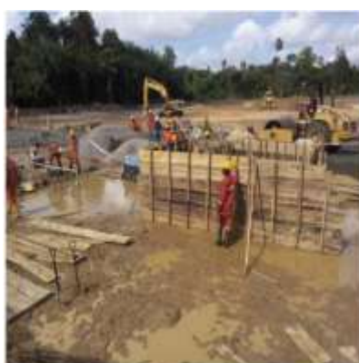
Septic tank construction/installation @Gbaran ubie protection works LNG-SPDC
