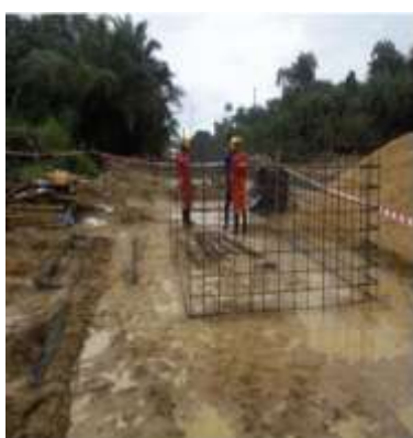
Septic tank construction/installation @Gbaran ubie protection works LNG-SPDC
