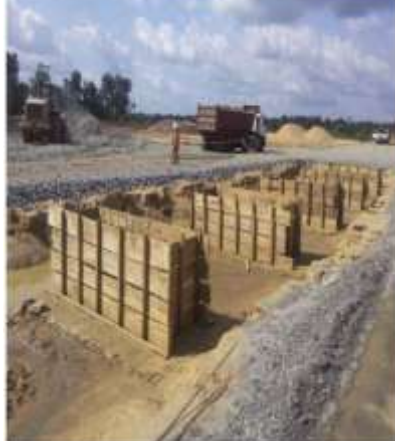
Weigh bridge foundation construction/installation@Gbaran ubie protection works LNG-SPDC
