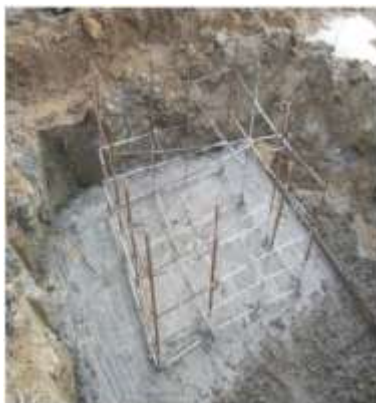
Mast foundation/erection @Gbaran ubie protection works LNG-SPDC
