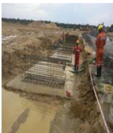
Weigh bridge foundation construction/installation@Gbaran ubie protection works LNG-SPDC
